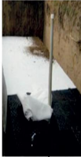
10. Leveled Surface after backfill
