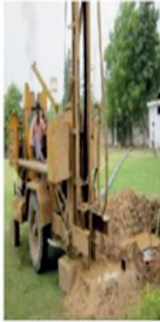
1. Recharge Well Drilling
