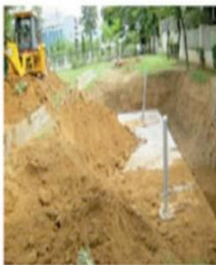
9. Backfilling Post Installation
